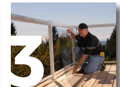
INSTALL PICKETS OR TEMPERED GLASS PANELS
