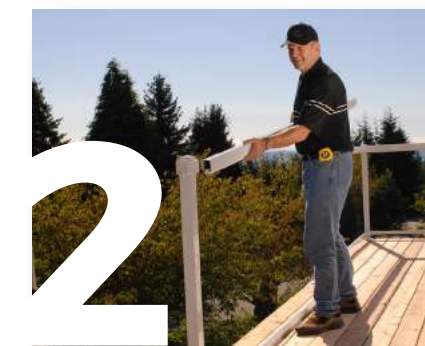
INSTALL TOP & BOTTOM RAILS
